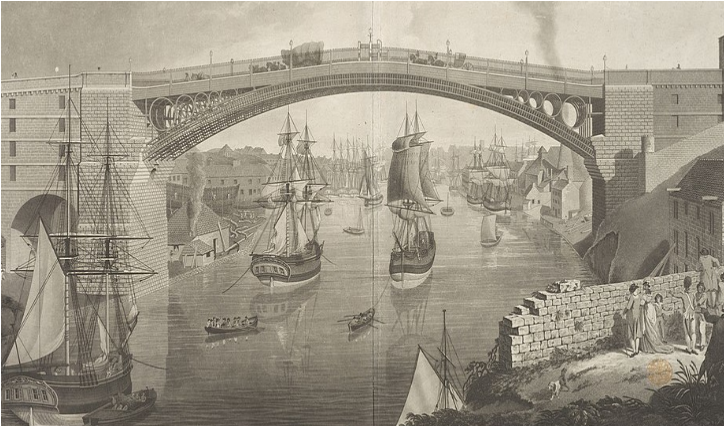
The Sunderland Bridge, above (from an engraving in Richardson's Table Book), used Thomas Paine's design as well as many of the cast-iron components first produced for Paine's "London Model" bridge. Paine went uncredited for his contributions.
